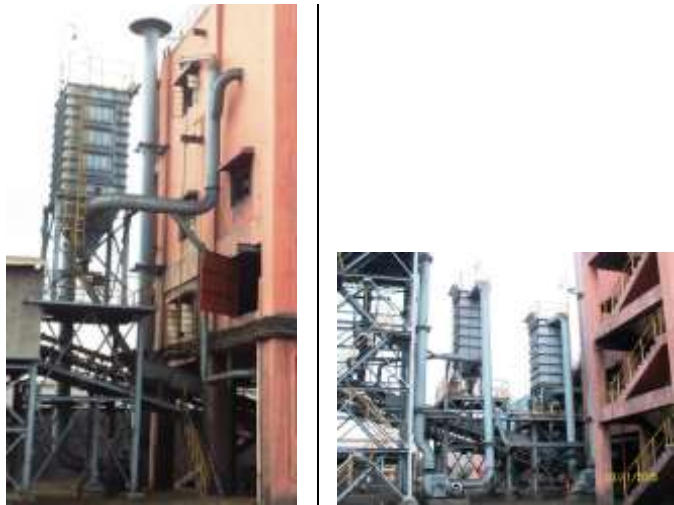
Dust Extraction System at CHP
